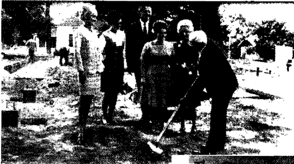
GROUND BREAKING — James Hammond, Sr., was the star of yesterday's groundbreaking for the new Union Safe Deposit Bank to be constructed in Lockeford. Watching the new
