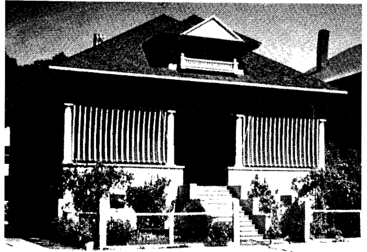
The new restaurant occupies the site of some apartment buildings the Wong family owned and the parking lot was the site of their old family home- Courtesy of the Wong family
